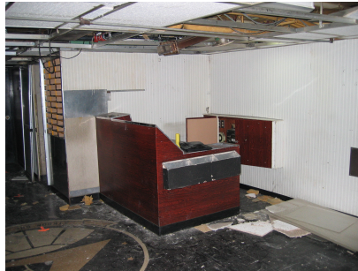
RR5 before clean-up.
